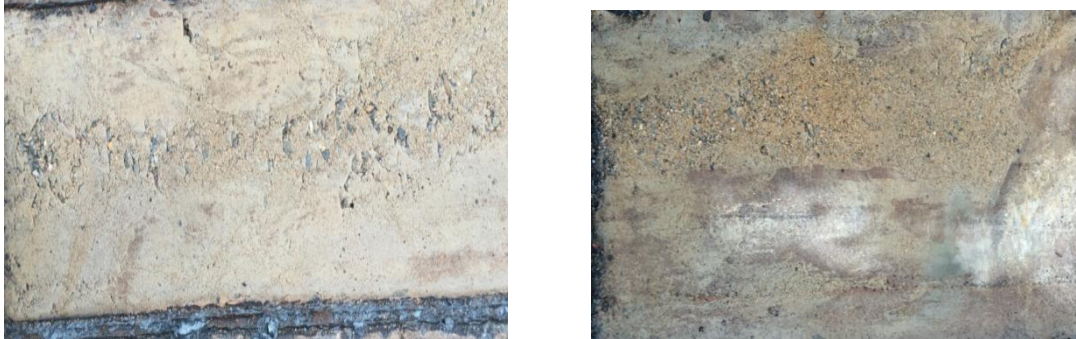
(a) honeycomb at 0.2-1m from the top of the member (b) honeycomb at 3-3.5m from the top of the member
